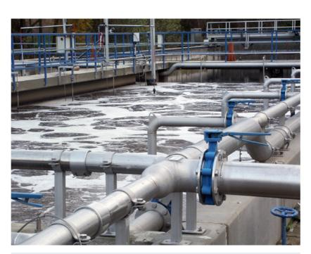
Aeration (wastewater treatment plant) Continuous recording of air flow for aeration of the activated sludge basin.
