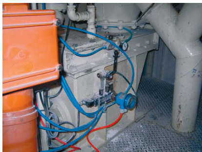
Mounting location of the Soliphant T
