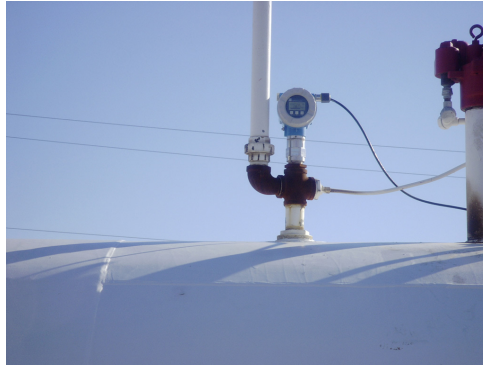
Levellflex FMP40 mounted in vent pipe on top of cylindrical fuel tank. Coax probe does not interfere with venting capabilities.
