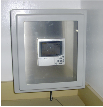
Ecograph T mounted in cabinet inside operators building
