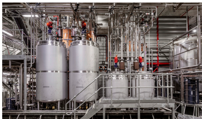
Maceration tanks with Endress+Hauser Micropilot FMR52 for level monitoring and control
