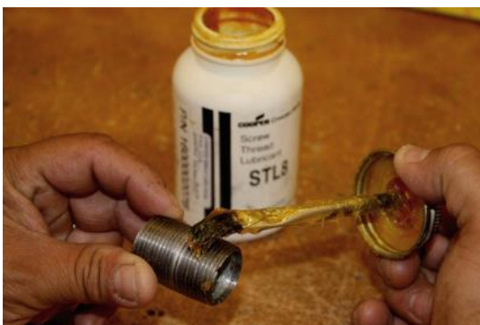
Figure 25. Applying lubricant to threads
