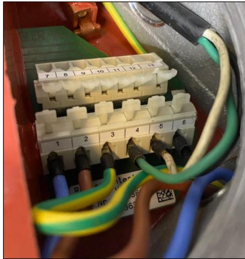
Fig 15. AC connection terminal block for enclosure heater
