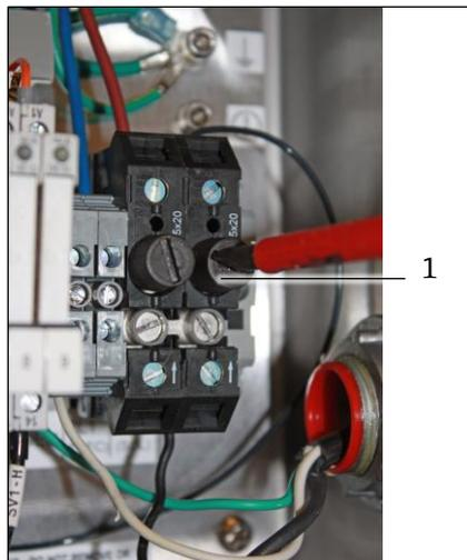
Fig 30. Unscrewing a fuse cover (1)
