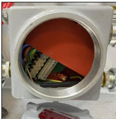
Fig 14. AC connection terminal block for enclosure heater
