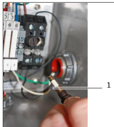
Fig 31. Replacing a fuse (1)
