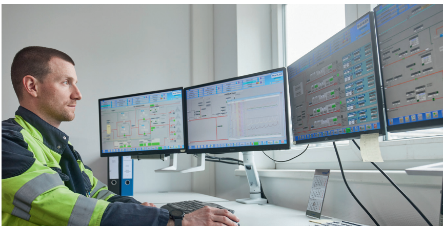
Out of the control room, Florian Wagner can check the verification of the pressure gauges.
