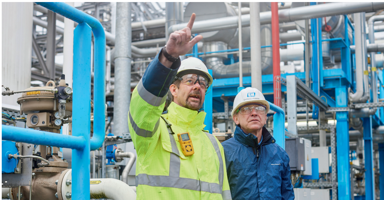
Plant manager Guido Kniepper with an Endress+Hauser employee in the hydrogen production plant.
