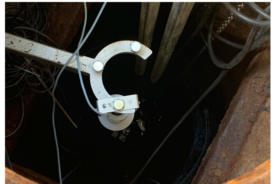
Multiple obstructions can often obscure the path of a radar. With a Bluetooth® operated mapping function, these can be easily removed.
