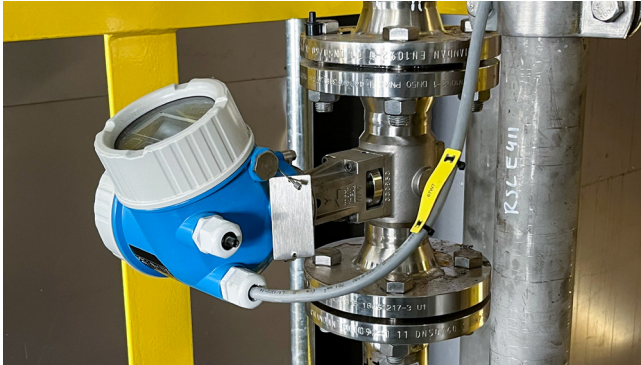
Vortex Flowmeter Proline Prowirl F200 for measurement of steam flow
