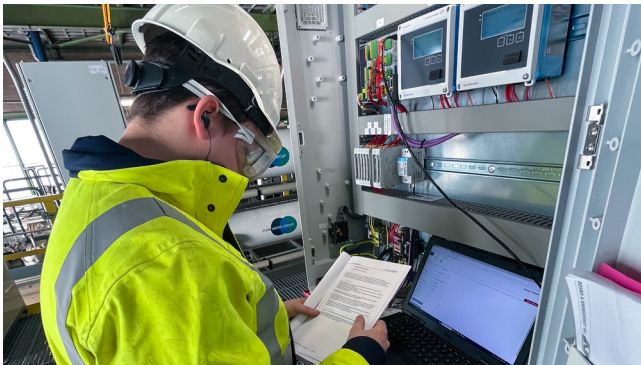
Endress+Hauser Service Engineer commissioning Energy Calculator EngyCal RS33 for steam and EngyCal RH33 for liquids together with Data Manager Memograph M RSG45
