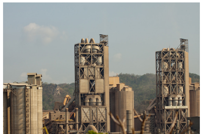
Example of a cyclone for preheating raw material
