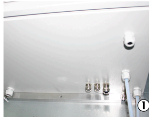
①. Sample gas outlet at rear of the housing (bottom view)
