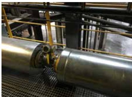
↑ Hydrogen measurement at the blast furnace with Prowirl vortex flowmeter plus Cerabar S pressure meters
