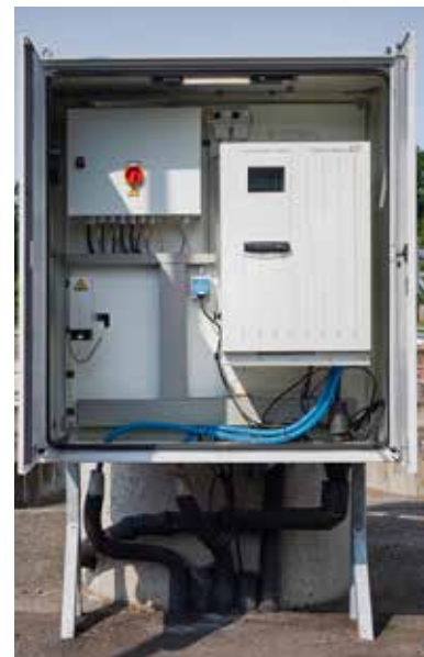
↑ The enclosure protects the analyzer from external influences
