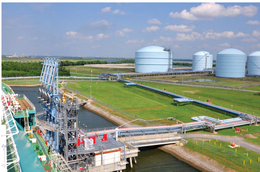
Aerial view of LNG facility
