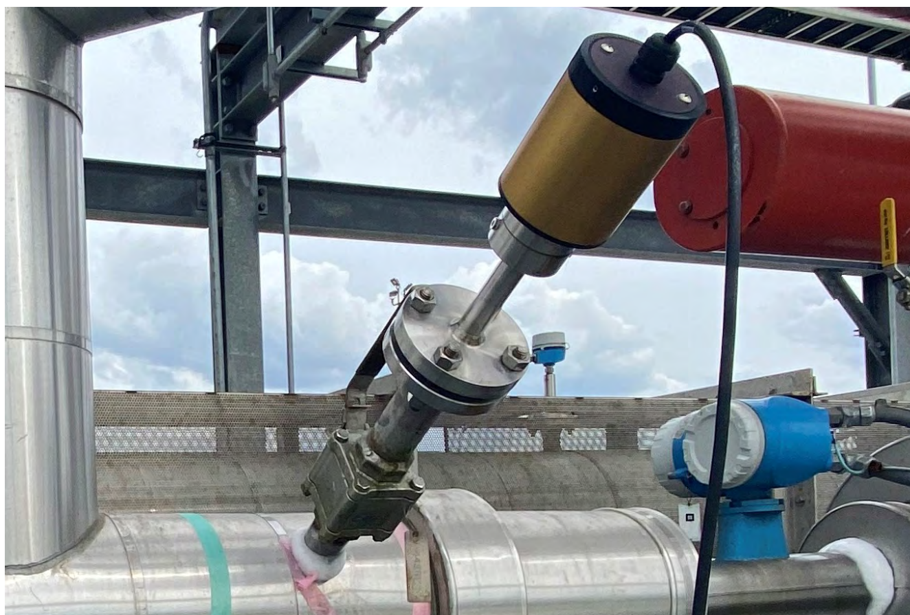
Raman Rxn-41 cryogenic probe with pigtail
