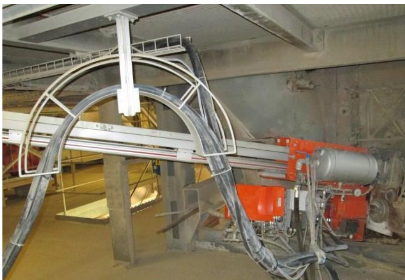
Fig. 30: Hose support mounted on the ceiling (example)
