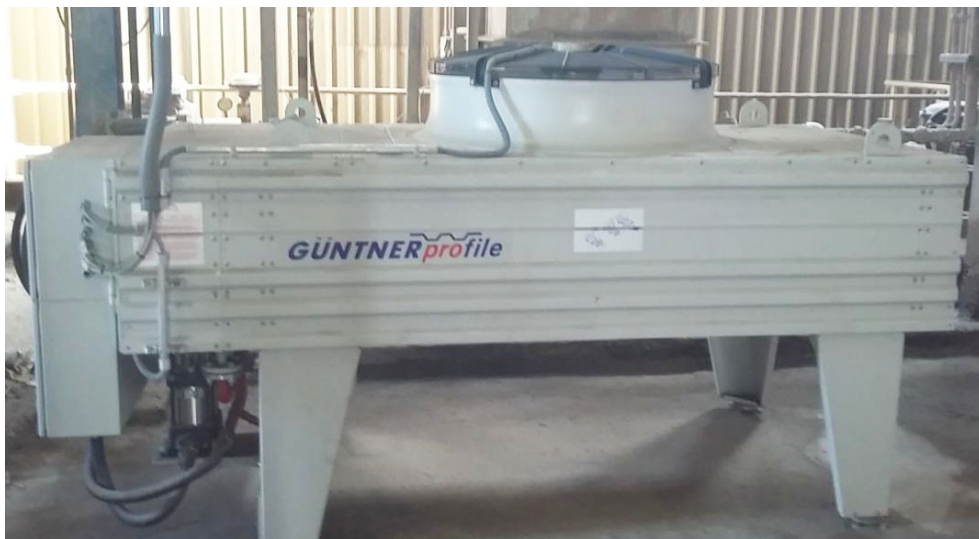
Fig. 40: Water to air cooling unit, completely installed
