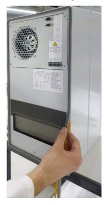
3 Attach cooling device to the cabinet and fasten 4 flange nuts.
