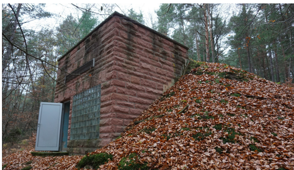
Spring tapping, reservoirs (discharge measurement)
