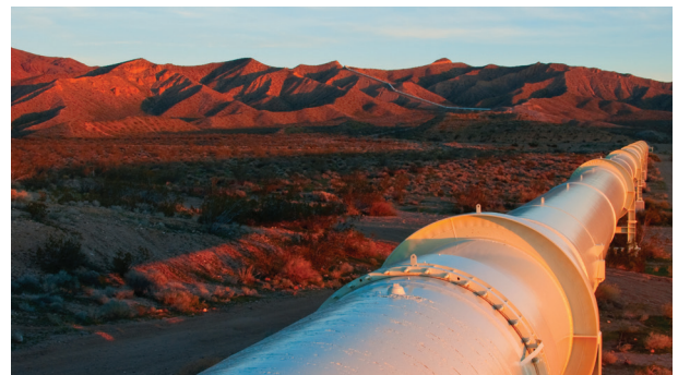
Transport pipelines (quantity measurement, leakage detection)
