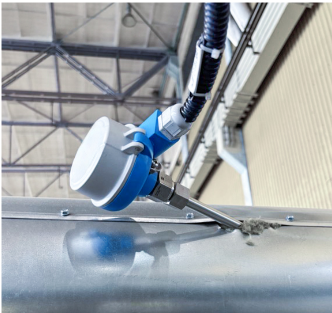
iTHERM SurfaceLine TM611 insulated in a cooling loop application
