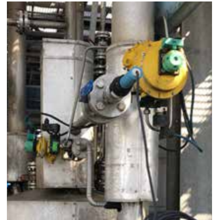
Oxygen measuring point with Memosens COS81D
