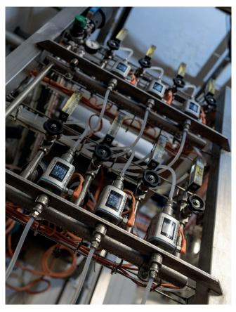
Thanks to the Picomag, tight installation spaces are no obstacle to ensuring precise flow measurements.
