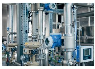
Every energy user is equipped with energy meters: Promag H electromagnetic flowmeters and temperature sensors monitor the mixer taps for the water that is used for the malt grinders.
