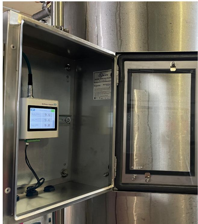
The transmitter of Teqwave H enables easy switching of recipes before a product change – directly in the plant or via laptop
