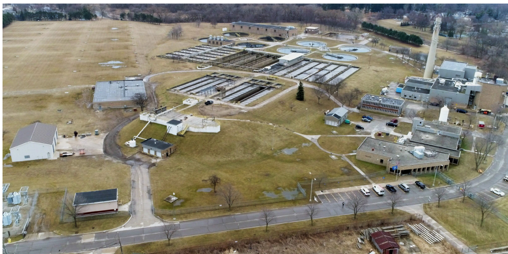
City of Warren Wastewater Treatment Plant
