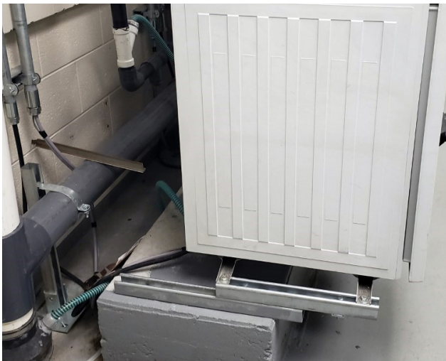
City of Warren samplers were built on tracks to allow the technicians and lab personnel ease of access to the process line and the back of the sampler.
