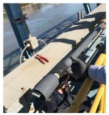
Turbimax CUS71D ultrasonic interface sensor immersed in clarified water mirror; assembly installation is carried out on the bridge of the thickener  $N^{\circ}2$
