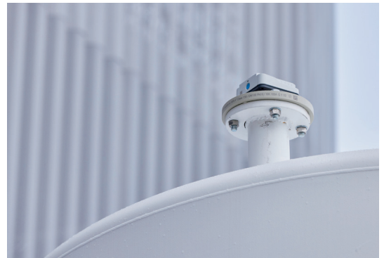
Sensor on silos: Level sensor Micropilot FWR30 (battery-powered)
