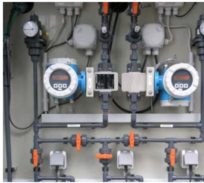
Compact installation of orthophosphate and total phosphorous analyzer CA80PH / CA80TP in the container (top)
