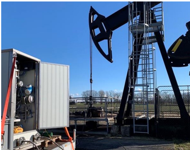
GPsol Wellchecker on a pumpjack
