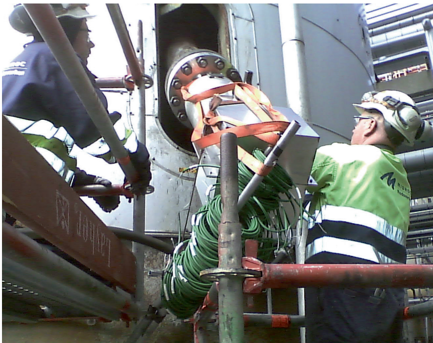
The iTHERM MultiSens multipoint assembly with 27 independent thermocouple sensors provides accurate temperature profiling in the reactor.
