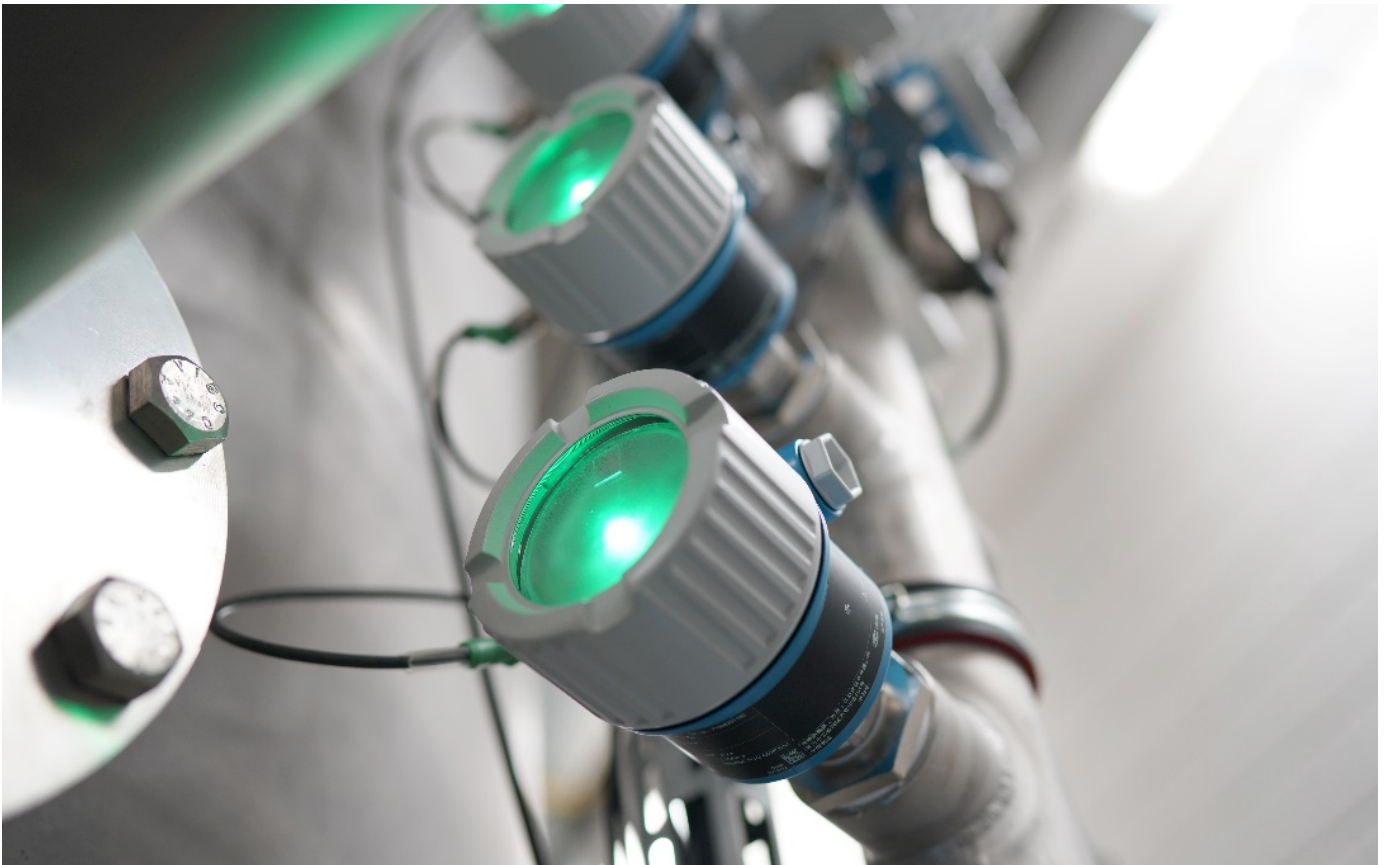
Figure 3: The Liquiphant FTL51B by Endress+Hauser, is SIL-rated, and can extend offline testing intervals with native online proof testing capabilities.
