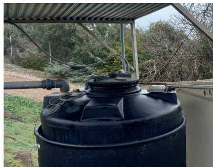
Sensor on silos: Level sensor Micropilot FWR30 (battery-powered)
