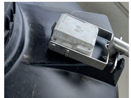
Sensor on silos: Level sensor Micropilot FWR30 (battery-powered)
