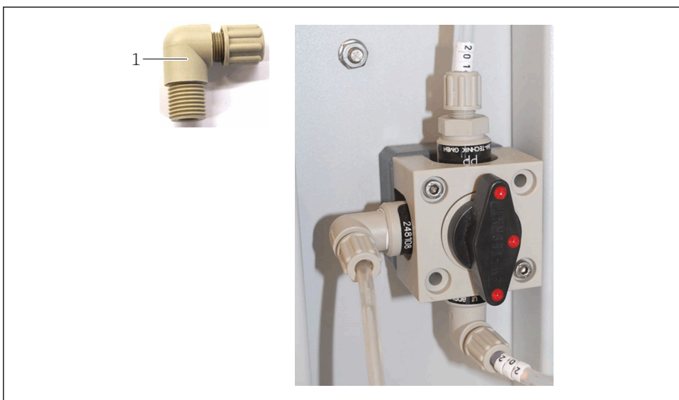
32 Angled coupling D 4/6 × G¼" PP on the sample channel switching
