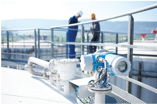
Figure 4: An accurate level instrument, such as this Endress+Hauser radar level transmitter, can detect when the level is dropping during inactivity, indicating a leak or spill
