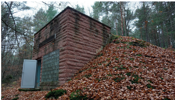
Spring tapping, reservoirs (discharge measurement)
