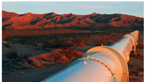
Transport pipelines (quantity measurement, leakage detection)
