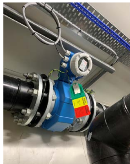
Conductivity sensors and flow assemblies installed to monitor the efficiency of salt removal in RO (left) and one of the many Promag P 300 electromagnetic flowmeters (right).
