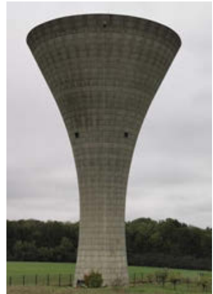
Redlach potable water reservoir (900m 3 )
