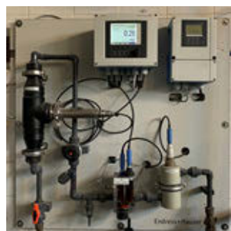
Analysis panel for measuring free chlorine at the end of the potable water treatment process
