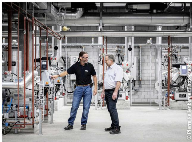
View into the energy center in the basement of the arena. Here, the cold for the ice rink, the air-conditioning cold for the dehumidification of the room air and the cold for surrounding office buildings are generated.
