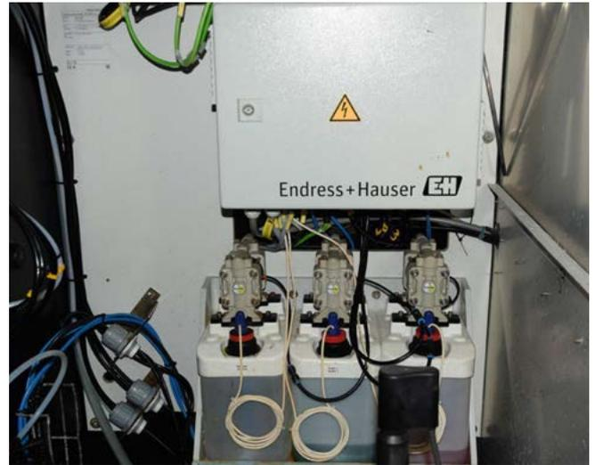
Liquiline Control CDC90 (photo left) and the pneumatic unit for automated supply of cleaning and calibration fluids (photo right).
