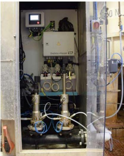
Liquiline Control CDC90 in the background in a case, with two pneumatically controllable retracting fittings for pH sensors on the front.
