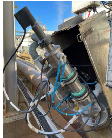
Ideal for heavy-duty applications: The pH retractable assembly CPA473
