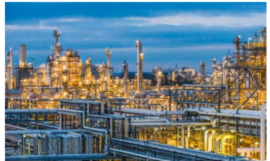
Basic and specialized chemicals are produced at the Dow plant in Stade, Germany.
