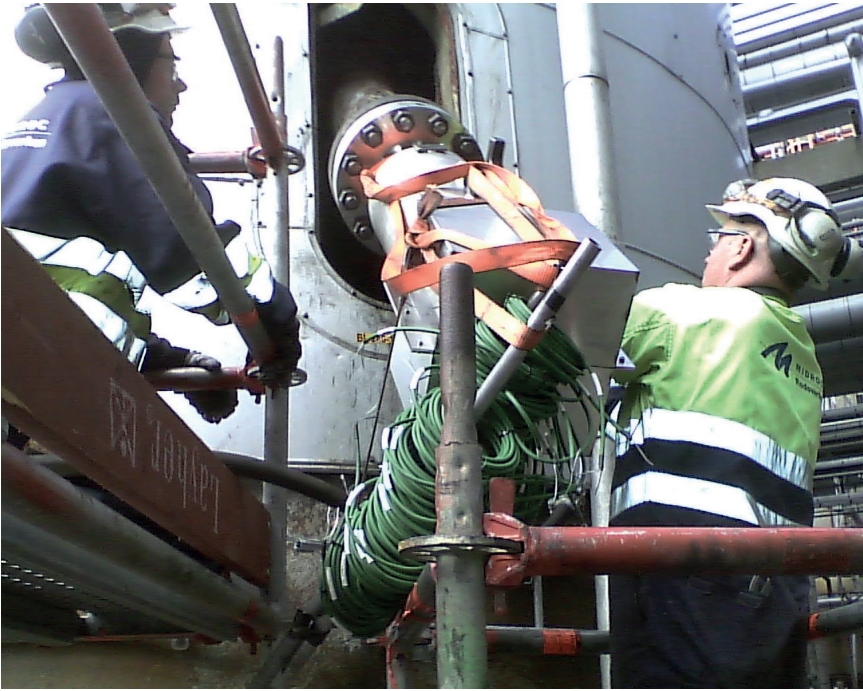
The iTHERM MultiSens multipoint assembly with 27 independent thermocouple sensors provides accurate temperature profiling in the reactor.
