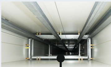
Insulating wall 1: around the water tank elevator
