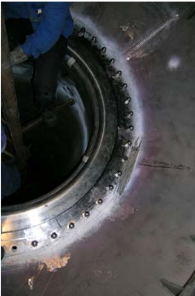
Mounting of iTHERM MultiSens Flex TMS02
