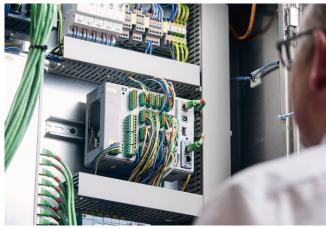
Industry 4.0 built into the switch cabinet: the Memograph M, with integrated web server, provides operators remote access for calling up stored data or configuring instrument parameters.
