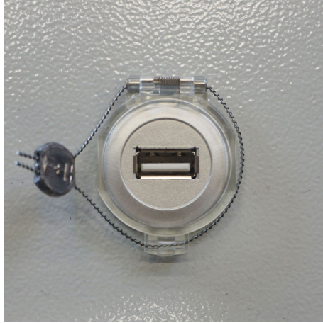
28 USB port sealed with sealing wire
