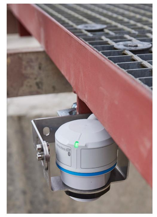
Device identification during Bluetooth connection thanks to "It's me-function" (LED flashing) and status indication via LED.
