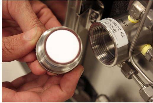
Figure 39: Inspecting the membrane separator filter
