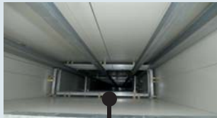
Insulating wall 1: around the water tank elevator
