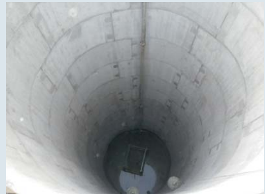
Insulation wall 2: Outside of insulating wall 1, vertical shaft in the underground part. Forced circulation inside each insulating wall
