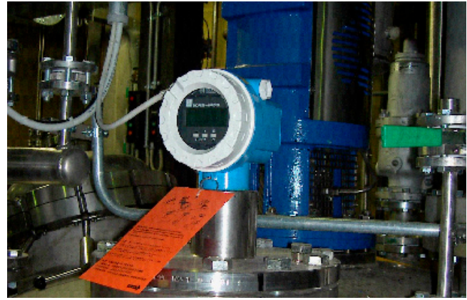
FMR 230 installation on the tank roof
