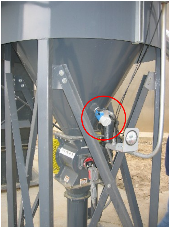
Soliphant II - FTM31 installed in a dust collection bin
