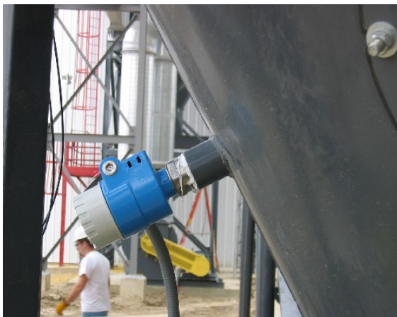
Mounting: Soliphant II - FTM31 installed in a full coupling
