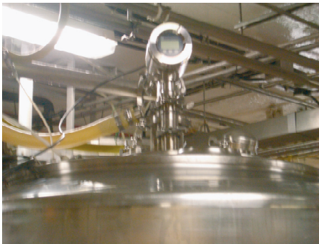
Levelflex M FMP40 on filler bowl
