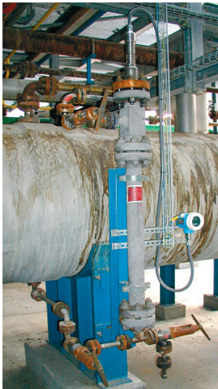
Levelflex M FMP45 installed in a bypass of a high temperature / high pressure application. The separate housing is used for easy access to setup the instrument.
