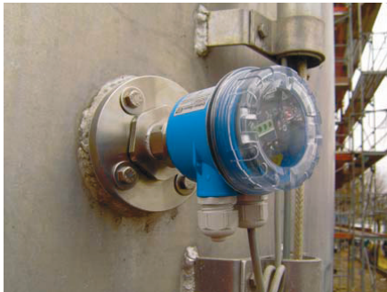
Mounting location of the Soliphant T
