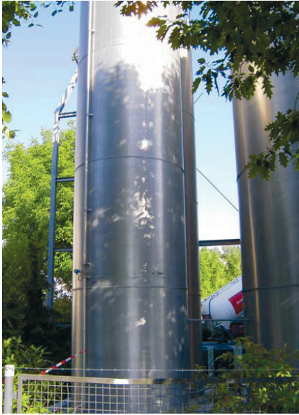
Solphant T FTM20 low level detection in a 33 ft high toothpaste powder storage tank triggers the re-order process when the material level is low.
